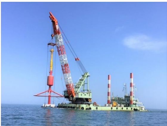
Installation of BuoyLidar (left), observations (right)
