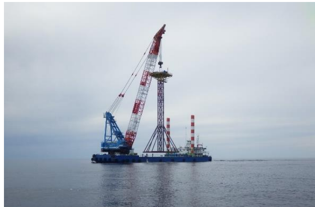
Seafloor survey (Installation of boring derrick by a crane ship)
